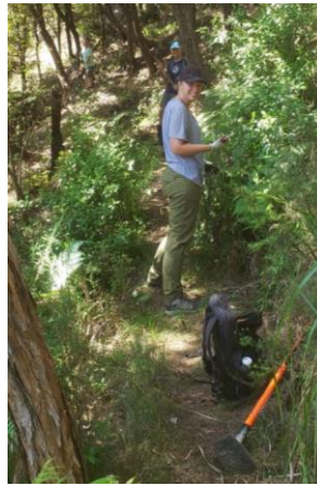
Re-benching and cutting back growth on the “Mawson ridge track”,
